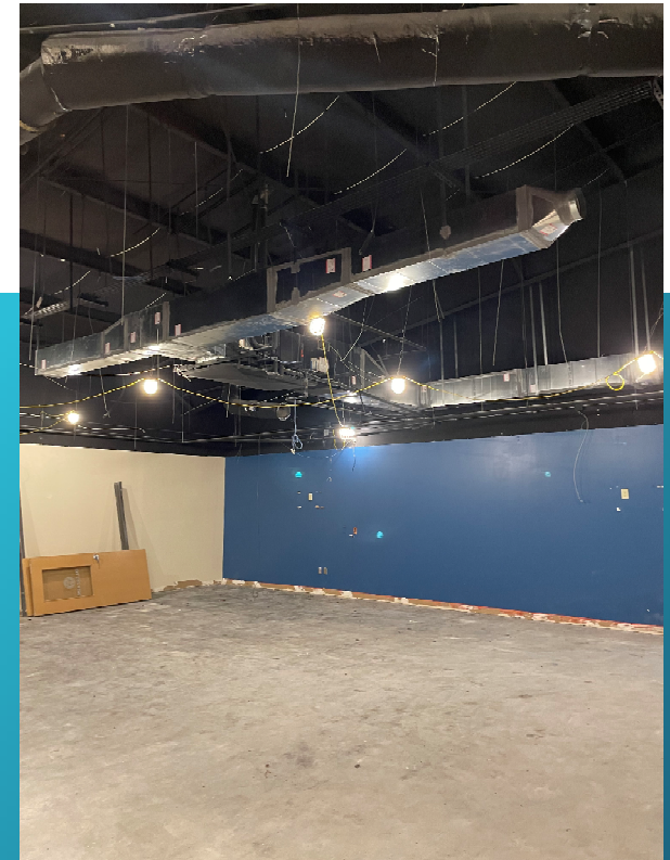
2 nd level Overhead Duct Work continues
