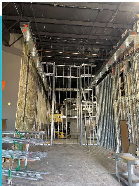
Chapel Framing and overhead ductwork
