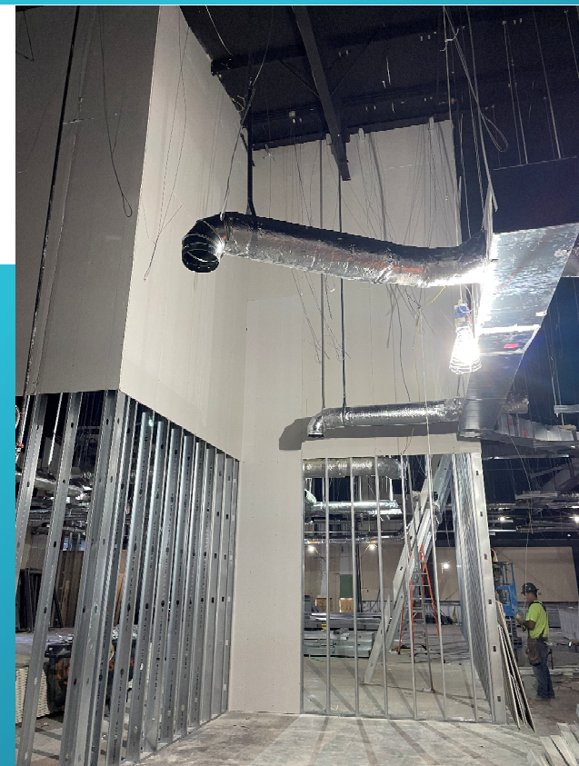
Sheetrock wall top out starting
