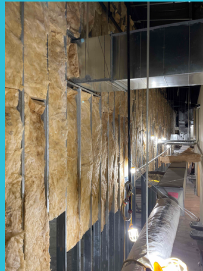
Insulation has Started
