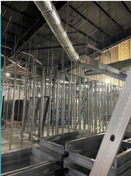
Door Frames Ready to Install
