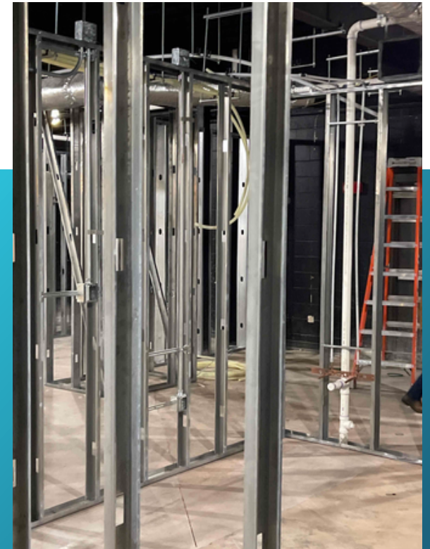
In wall Rough in Continues
