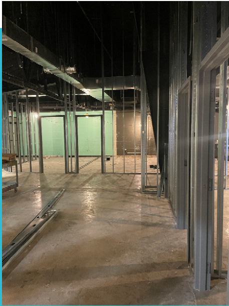
Door Frames Installed
