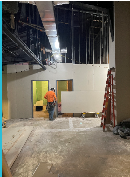
Hanging of Sheetrock walls full height
