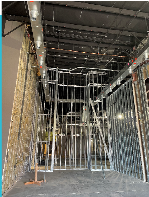
Chapel – Walls and duct installed
