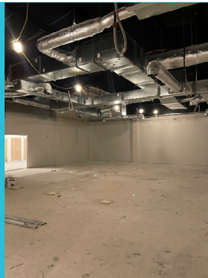
Duct Insulation being Installed
