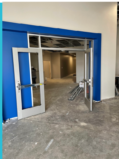
Aluminum Storefront Being Installed
