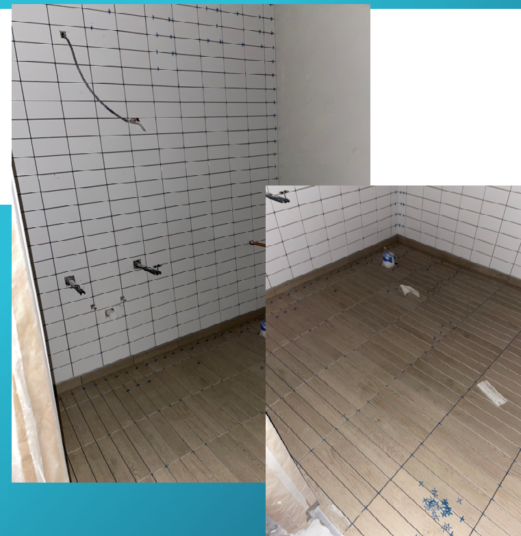
Restroom Tile Being installed
