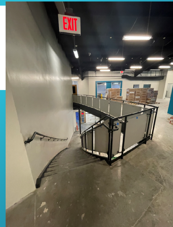
Handrail screening re-installed
